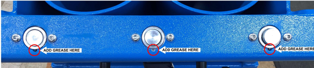
Figure 5.1: Location of grease points in top of fill door.
